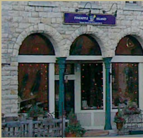
Maintenance of original Pilasters
