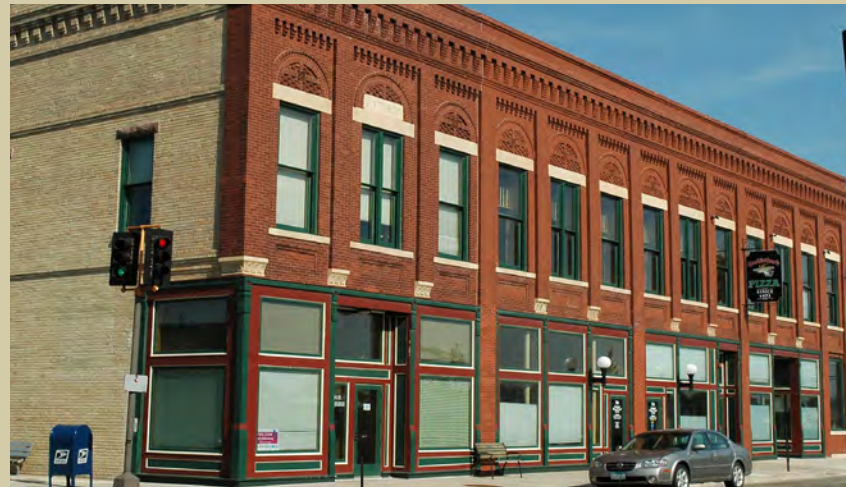
Continuity between multiple entrances.
