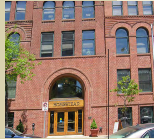
Masonry matches historic Style but mortar does not
