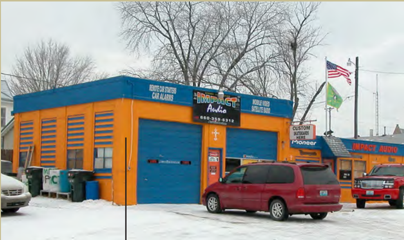
Bright, bold colors are inappropriate for traditional commercial buildings within the Plattsburgh Historic District
