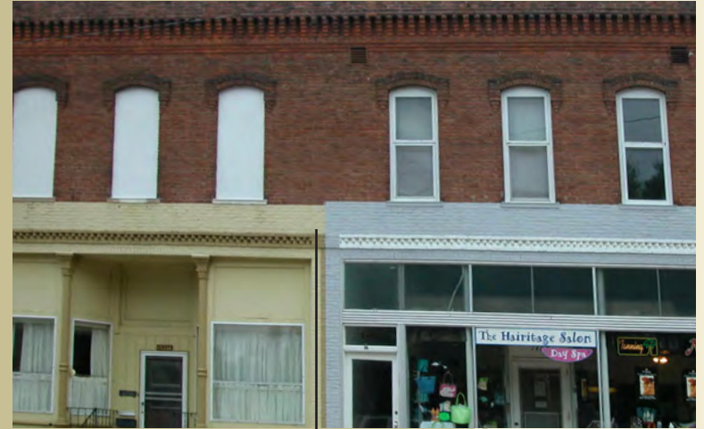
Avoid painting originally unpainted brick and maintain continuity between lower and upper floors
