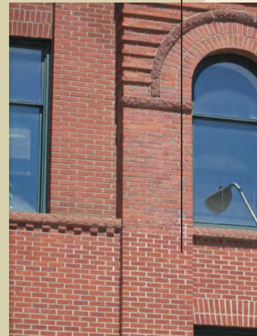
Masonry matches historic Style but mortar does not
