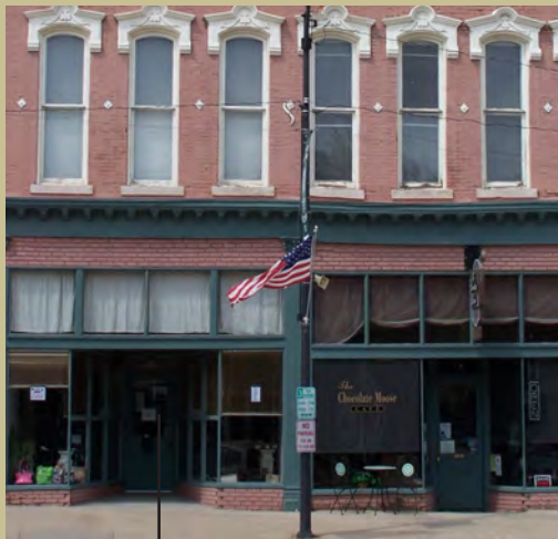
Rehabilitation of original entrances
