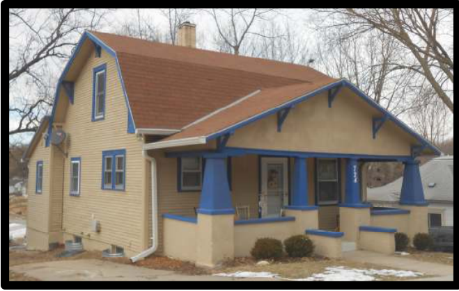
Figure 8: Photograph by APMA December 2013.
