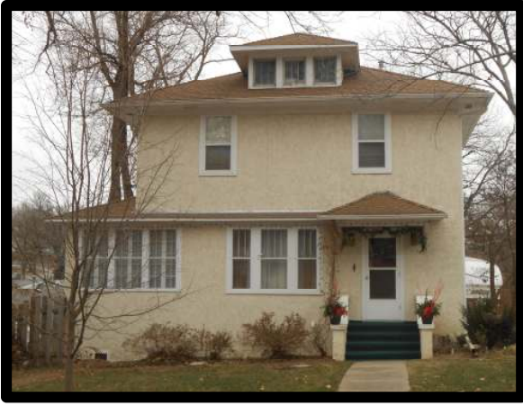
Figure 12: Photograph by APMA December 2013
