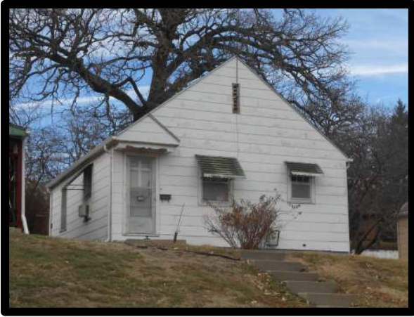
Figure 16: Photograph by APMA December 2013.
