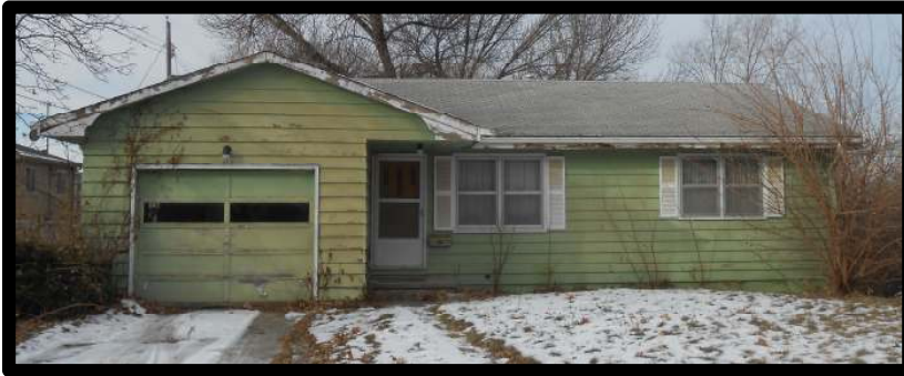
Figure 21: Photograph by APMA December 2013.
