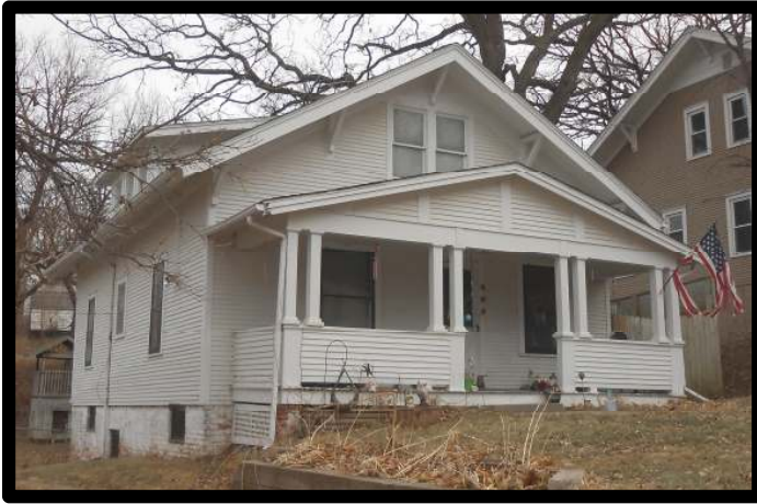
Figure 9: Photograph by APMA December 2013.
