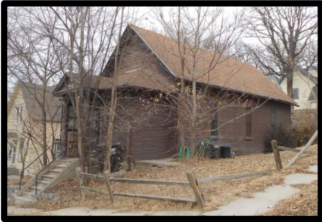
Figure 22: Photograph by APMA December 2013.
