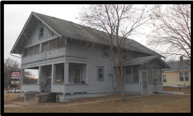
Figure 11: Photograph by APMA December 2013
