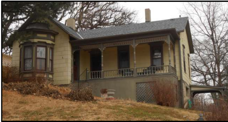
Figure 26: Photograph by APMA December 2013.
