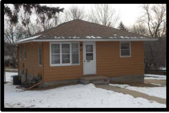
Figure 17: Photograph by APMA December 2013.
