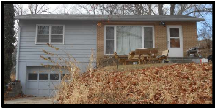
Figure 20: Photograph by APMA December 2014.
