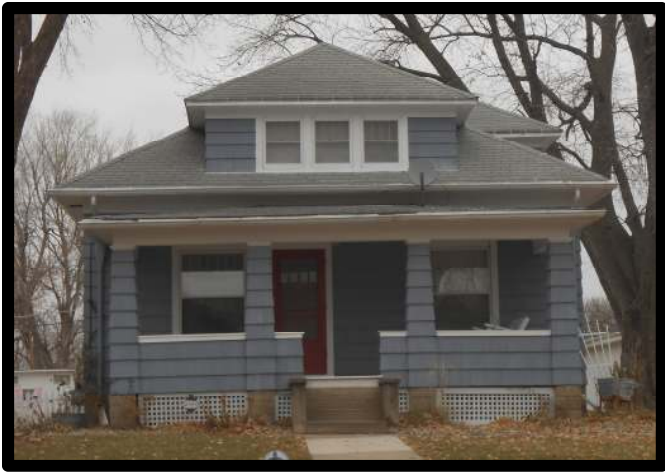
Figure 7: Photograph by APMA December 2013.
