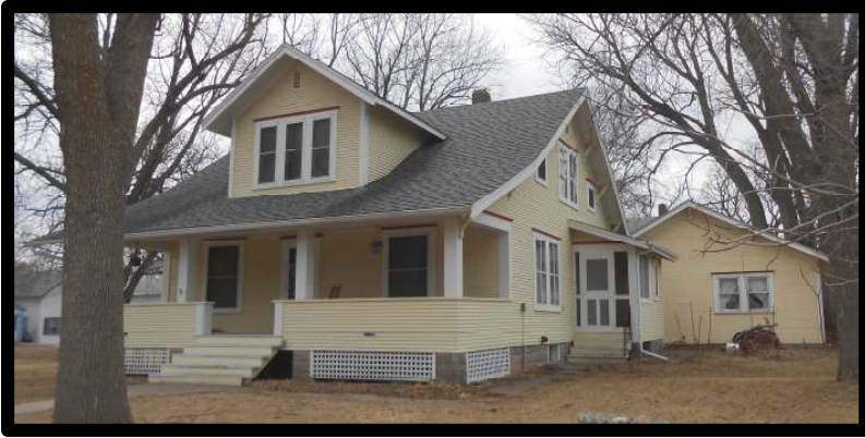
Figure 10: Photograph by APMA December 2013
