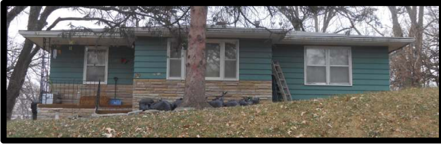
Figure 18: Photograph by APMA December 2013.
