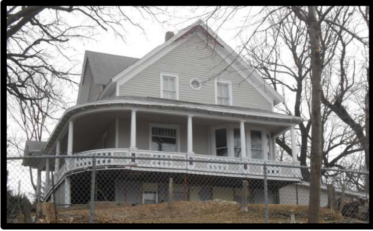
Figure 6: Photograph by APMA December 2013.
