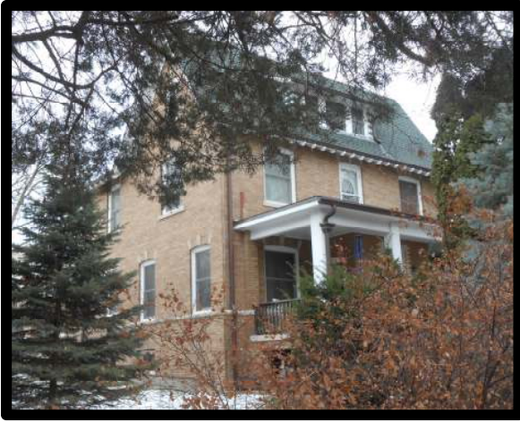
Figure 13: Photograph by APMA December 2013.
